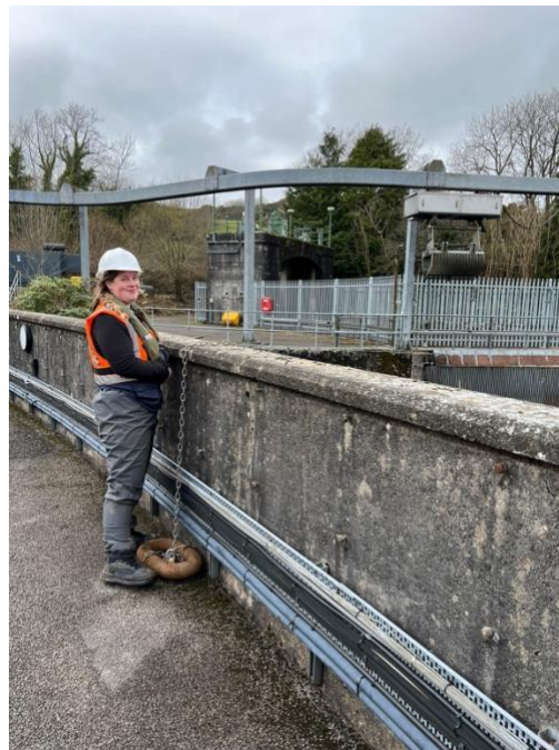
Deploying acoustic receiver at Tongland Dam
